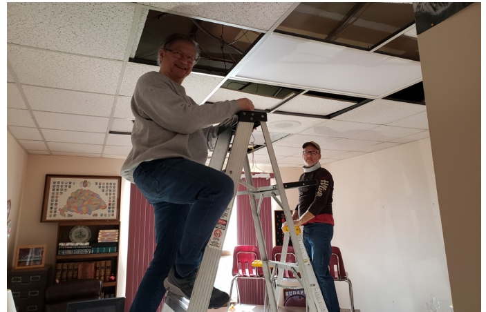
Dr. Albert Ladanyi Chief Elder and John Janosik Trustee replace the old fluorescent lights to new LED light fixtures
