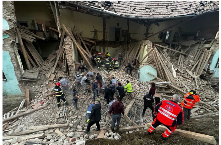
The collapsed dormitory of the Tamási Áron Roman Catholic High School, Székelyudvarhely
